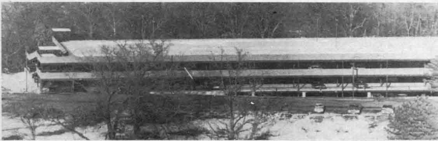
TOWERING VIEW: The expensive, new garage eases the search for parking spaces, while cars without shelter use
